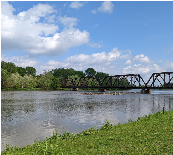
Figure 14: Railroad bridge to Turkey Island
