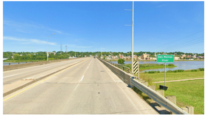
Figure 63: Existing Wapello Street Bridge
