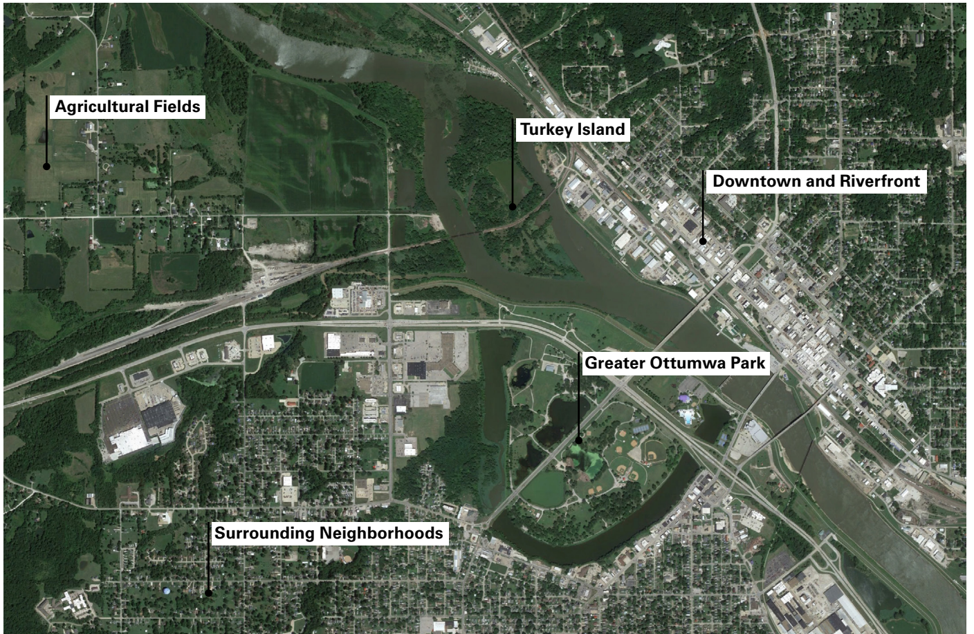
Figure 13: Birds-eye view over the site to existing agricultural fields, neighborhoods, Turkey Island and downtown
