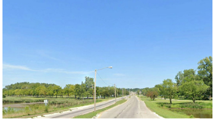
Figure 61: Existing Wapello Street
