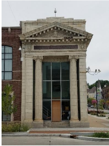
Figure 57: Non-original storefront system. South elevation. Sept. 2021.
