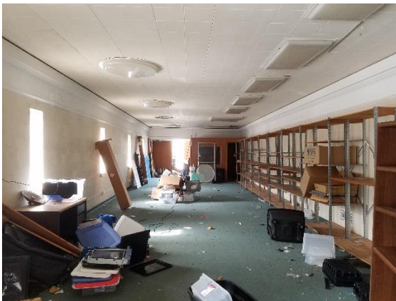
Figure 67: Overall view of first floor, view south. Sept. 2021.
