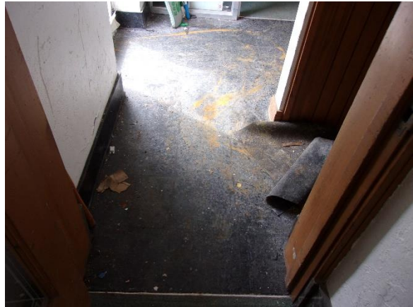
Figure 76: Tile flooring at first floor. Sept. 2021.
