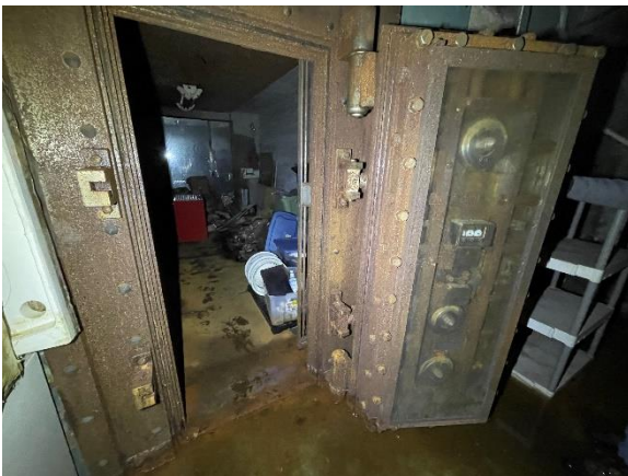
Figure 93: Vault at basement level.
