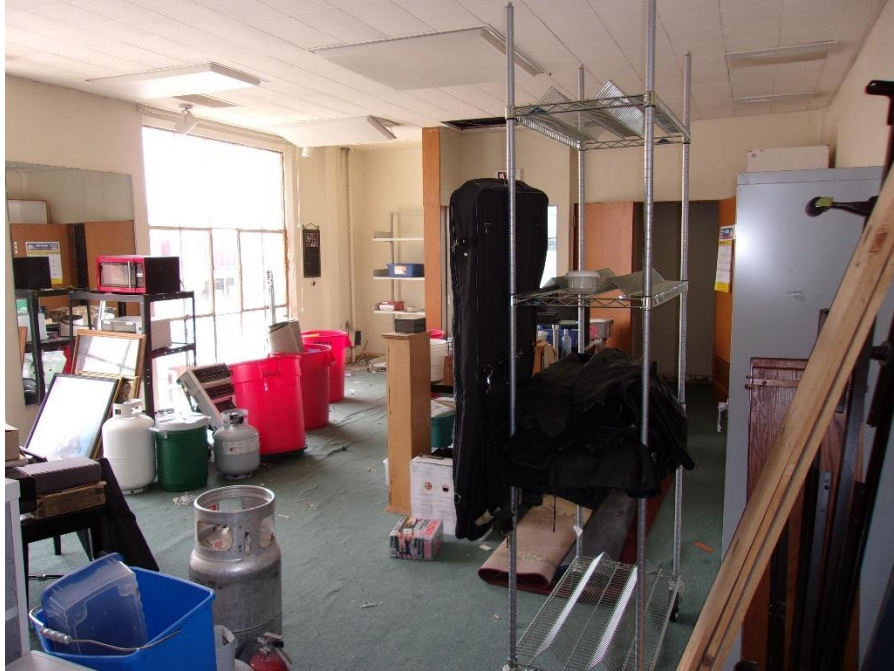
Figure 40: Typical second floor conditions, view southeast. September 2021.
