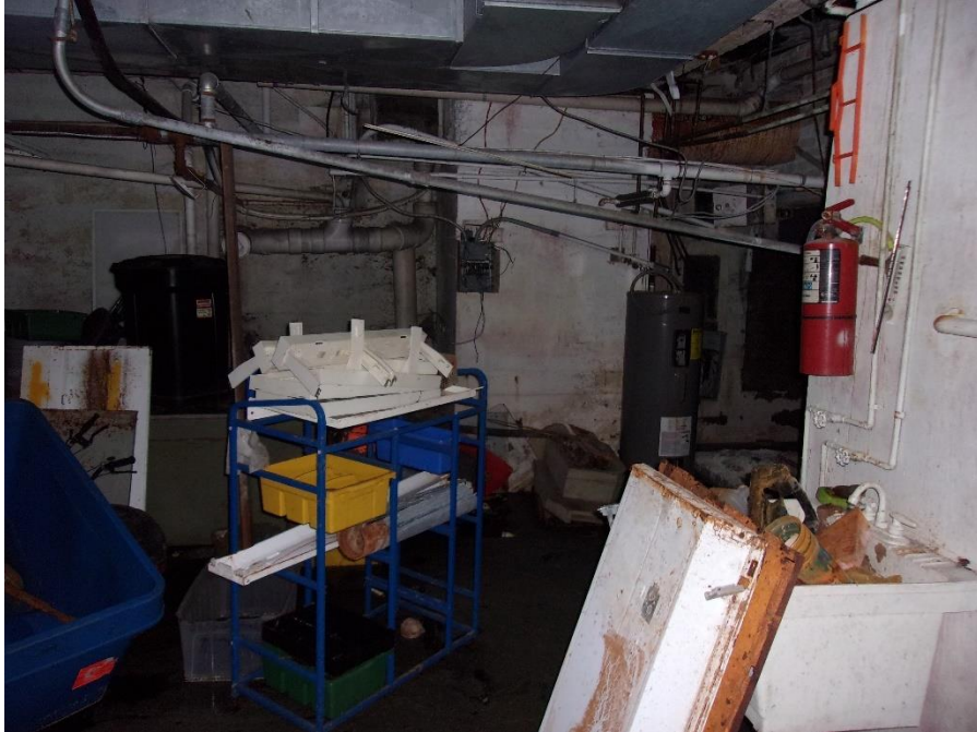
Figure 38: Typical basement conditions. September 2021.
