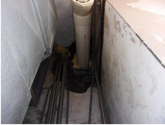
Figure 101: Plumbing pipes at second floor.
