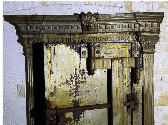
Figure 94: Vault at basement level.
