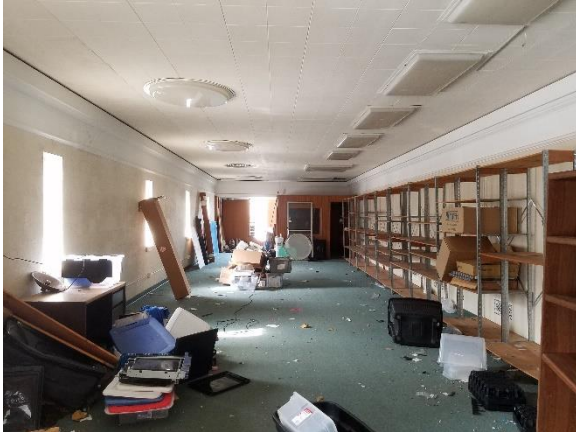
Figure 82: Typical ceiling at first floor. Sept. 2021.
