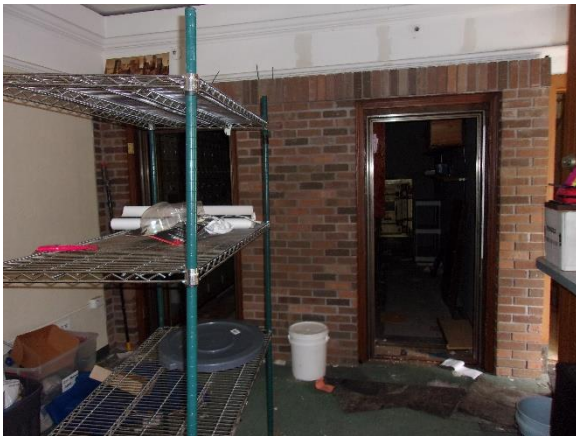
Figure 71: Brick veneer accent wall (not original), view north. Sept. 2021.
