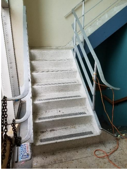
Figure 79: Terrazzo flooring (likely dating to 1956 remodel) at front entryway. Sept. 2021.
