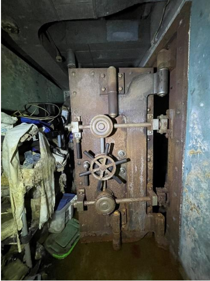
Figure 95: Vault at basement level.
