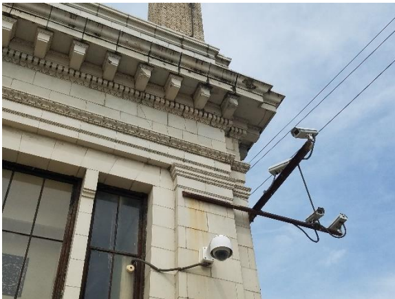
Figure 63: Security cameras at northeast corner. Sept. 2021.
