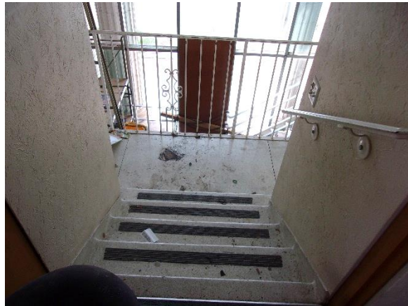
Figure 112: Steps from front entry staircase at second floor. Sept. 2021.
