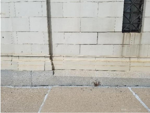
Figure 54: Typical condition of foundation wall, gray granite. East elevation. Sept 2021.
