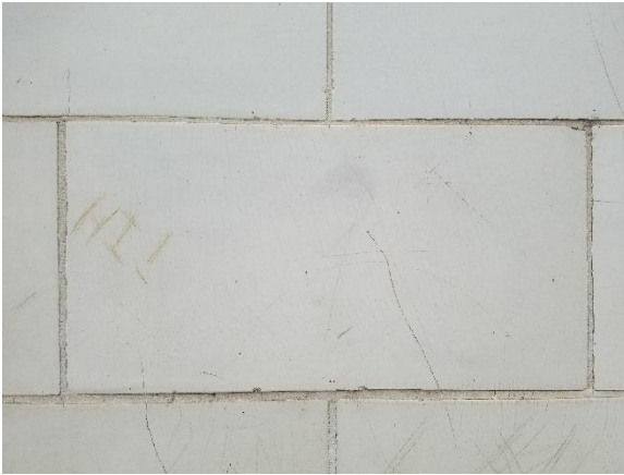
Figure 25: Terra cotta clad exterior walls, east elevation. Sept. 2021
