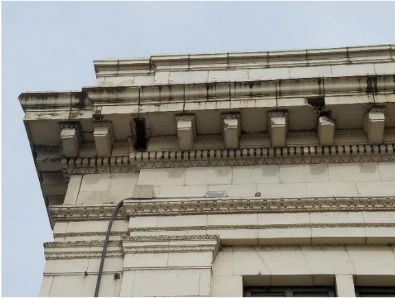
Figure 50: Typical cornice detail, east elevation. View west. Sept. 2021.
