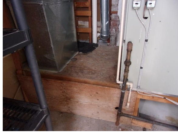
Figure 102: Plumbing pipes at second floor.
