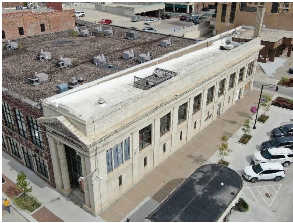
Figure 42: View of roof, view northwest. Sept. 2021.
