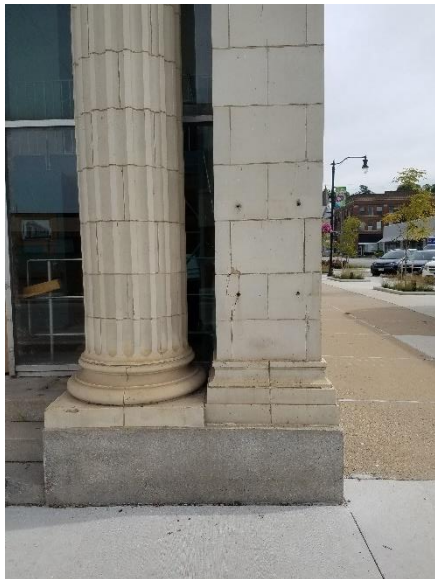
Figure 56: Typical condition of foundation wall, gray granite. South elevation. Sept 2021.
