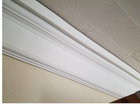
Figure 83: Cornice at first floor. Sept. 2021.
