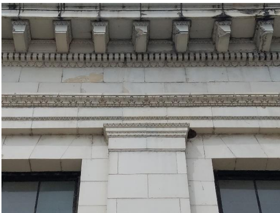
Figure 22: Trim and Secondary Features: Building features typical Neo-classical details such as modillions, acanthus leaves and lonic columns as part of the temple front. View west. Sept 2021.
