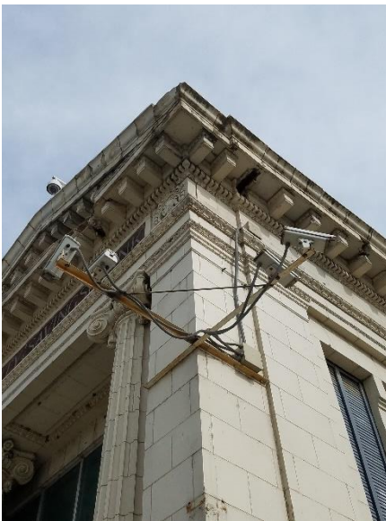
Figure 27: Terra cotta details at cornice, view northwest. Sept. 2021
