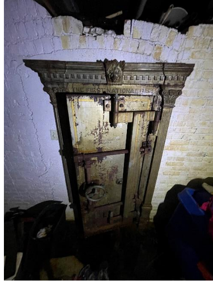
Figure 96: Vault at basement level.
