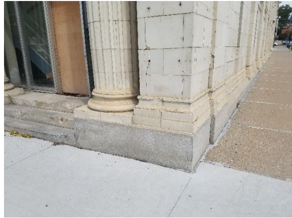
Figure 26: Stone and terra cotta exterior materials. Sept. 2021.
