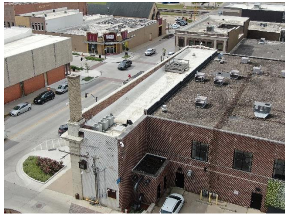
Figure 43: View of roof, view southeast. Sept. 2021.
