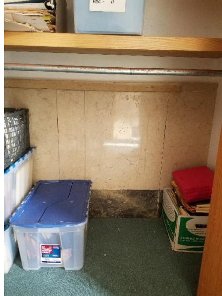
Figure 88: Original marble wainscoting at first floor. Sept. 2021.
