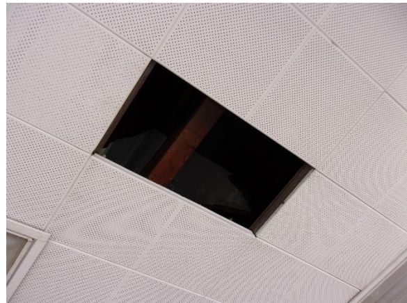
Figure 85: Typical acoustical ceiling tile throughout first and second floor. Sept. 2021.
