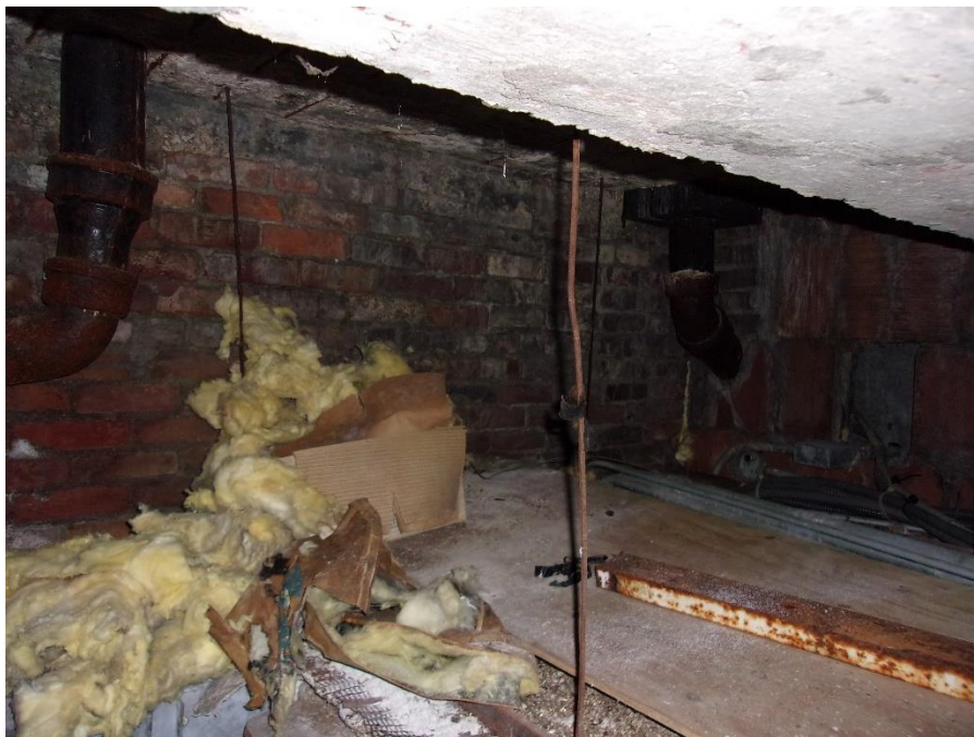
Figure 41: Typical attic conditions. September 2021.
