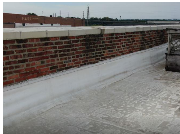
Figure 45: Back of parapet wall, view southeast. Sept. 2021.
