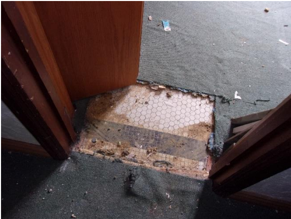
Figure 75: Original tile flooring at first floor. Sept. 2021.
