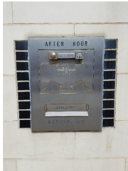
Figure 28: One of two after-hours drop box. Date of installation unknown. 2021.
