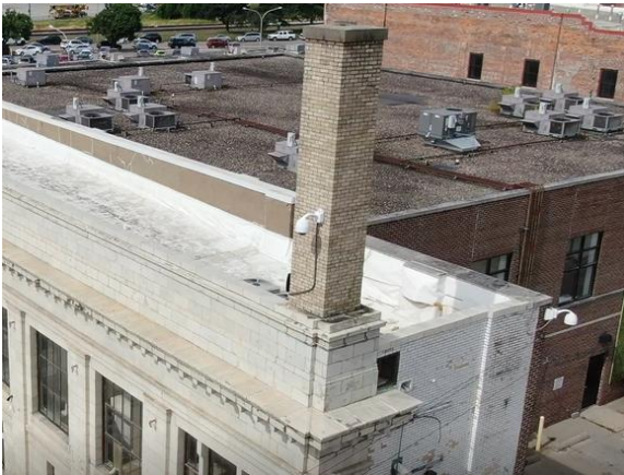
Figure 46: Chimney at north end of building, view southwest. Sept. 2021.
