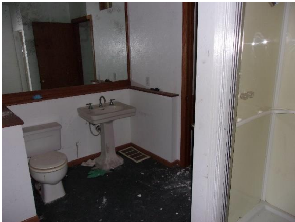
Figure 89: Typical bathroom fixtures (not original to building). Sept. 2021.
