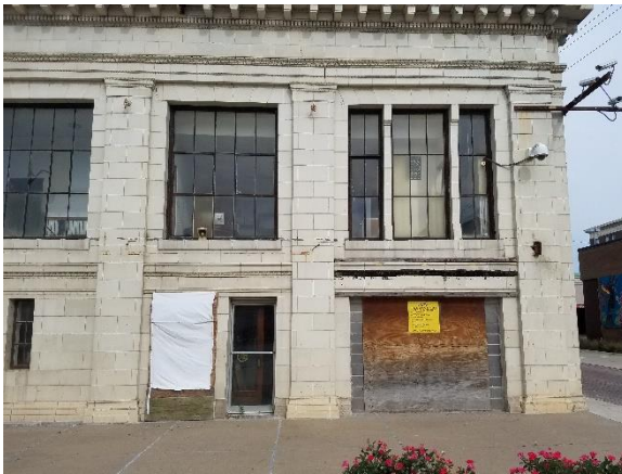
Figure 59: Typical window and door conditions. East elevation. Sept. 2021.
