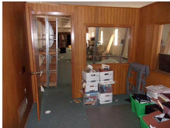
Figure 68: Interior view of office at first floor, view north. Sept. 2021.
