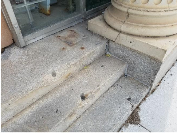
Figure 109: Three steps exist at south entry. Sept. 2021.
