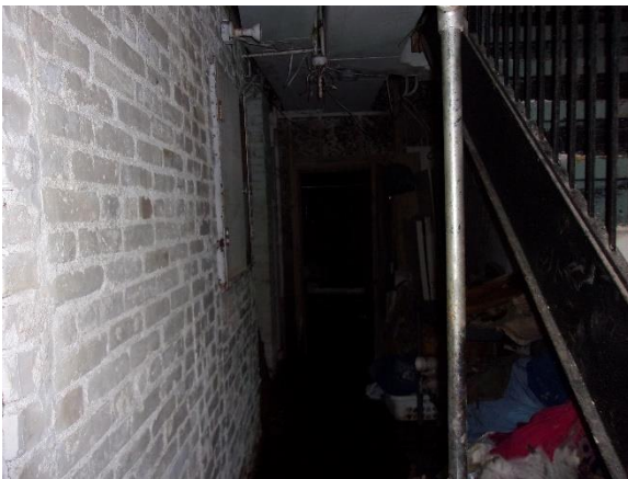
Figure 97: Basement foundation wall. Sept. 2021.
