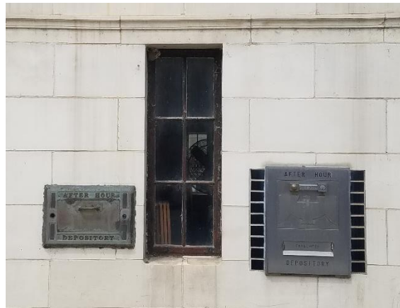
Figure 64: After hour deposit boxes located on east elevation. Sept. 2021.
