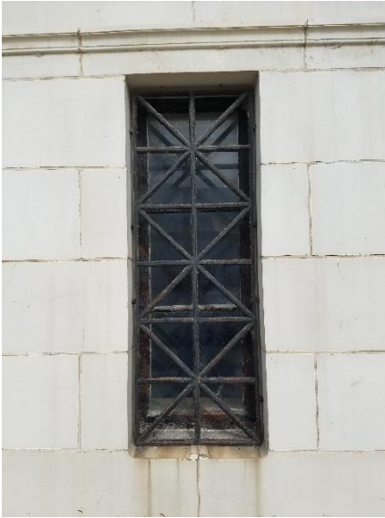
Figure 61: Typical first floor window, with security grille. East elevation. Sept. 2021.
