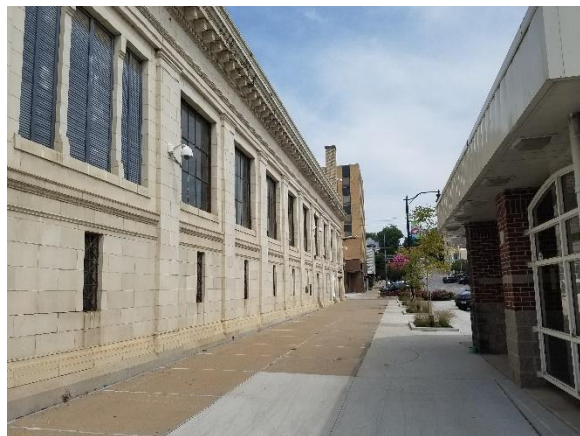
Figure 21: Projections: No projections protrude from the building beyond the cornice at this time. View north. Sept. 2021.
