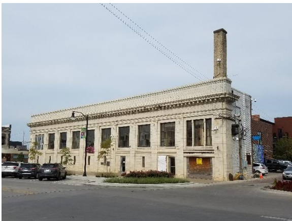
Figure 20: Openings: Openings are original and repetitive. View southwest. Sept. 2021.
