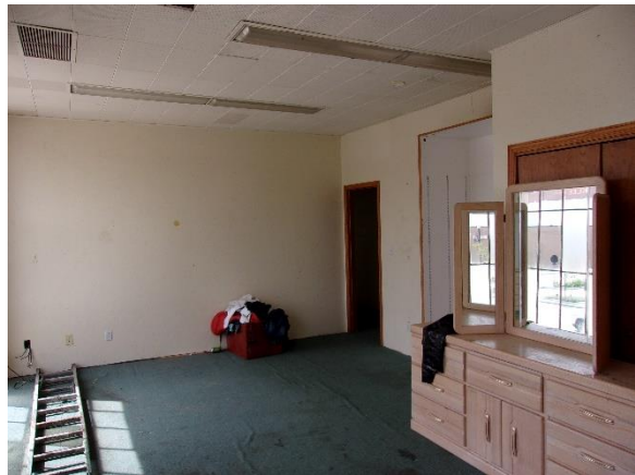
Figure 72: Typical walls at second floor. Sept. 2021.
