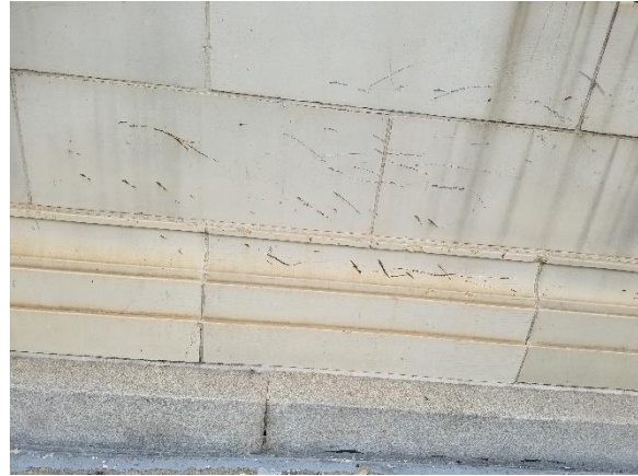
Figure 51: Base details at east elevation. View west. Sept. 2021.
