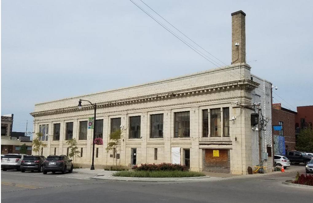
Figure 36: Overall east elevation. September 2021.
