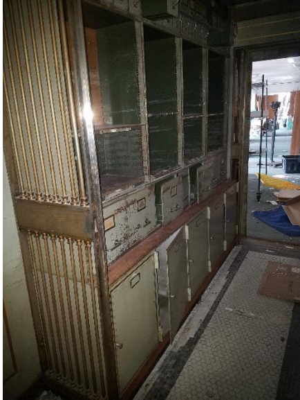
Figure 91: Vault furnishings, first floor. Sept. 2021.
