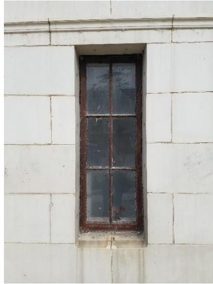
Figure 62: Typical first floor window, without security grille. East elevation. Sept. 2021.
