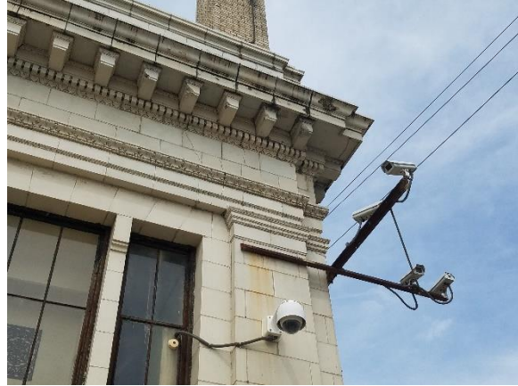
Figure 105: Security cameras at northeast corner. Sept. 2021.
