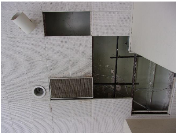
Figure 86: Original ceiling exposed above dropped ceiling at south entry. Sept. 2021.
