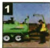
1 Clean area with on-board airstream
